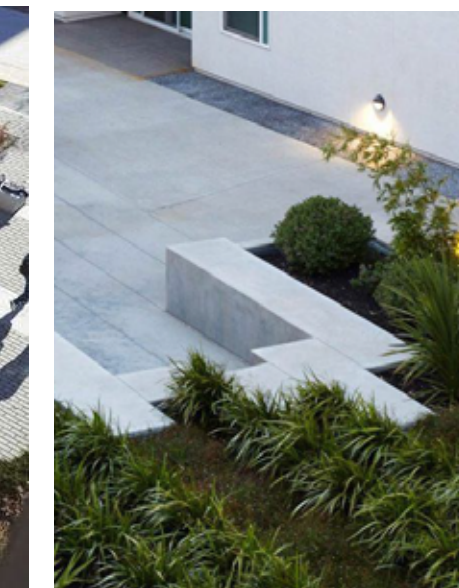
SEATING EDGES AS RETAINING
