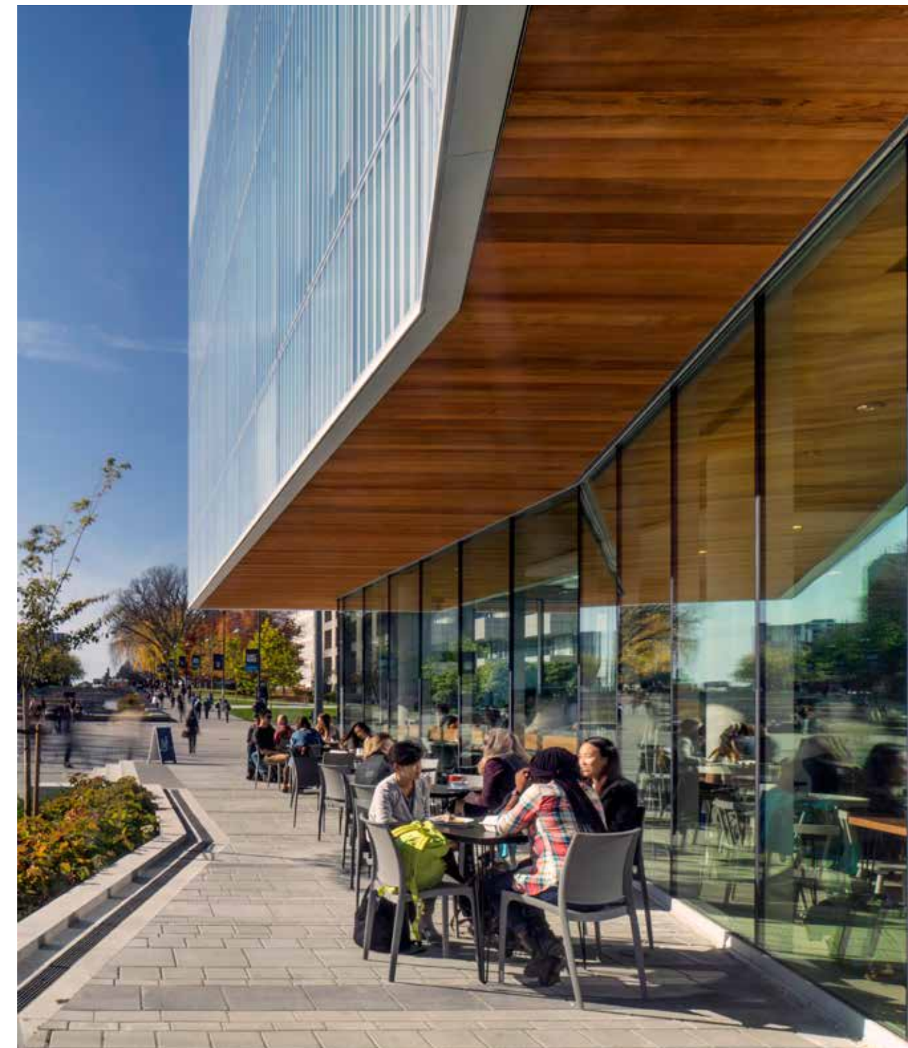
SSG Curtain Wall (with Cedar Soffits)
